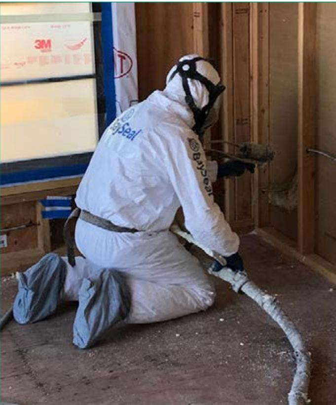
**Figure 5.** Because of the home's transportation and assembly requirements, as well as its need to dramatically reduce energy demands, the use of spray polyurethane foam proved ideal. SPF's unique properties are leveraged to join, seal, and waterproof the Flex House. Photo courtesy 951 Construction.
