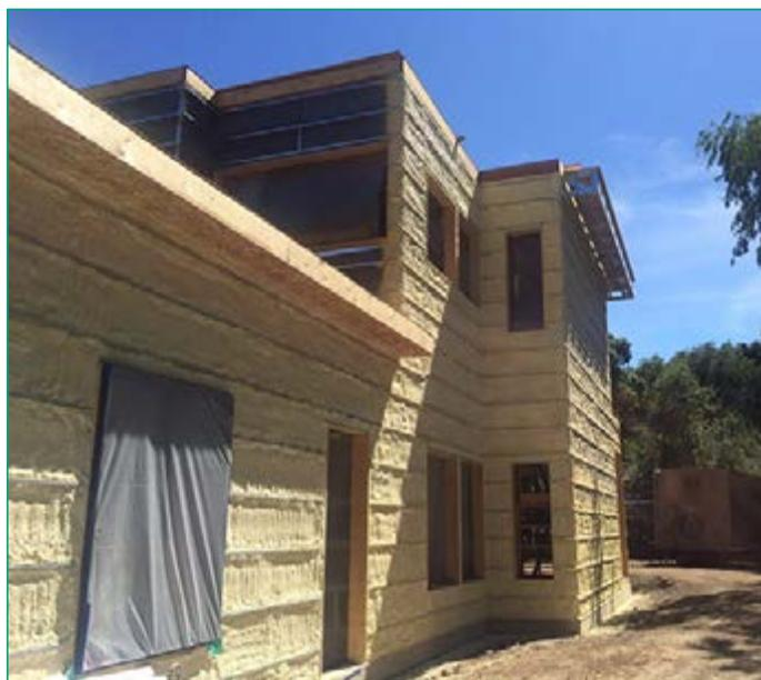
**Figure 3.** SDI Insulation, Inc., a Northern California insulation contractor, completed all spray polyurethane foam applications in the home. SDI applied Accella BaySeal open cell spray foam in the underside of the roof panels as well as Accella BaySeal closed cell spray foam to the outside of the exterior walls, providing extra R-value, air sealing and structural strength, while creating a rain screen between the spray foam and the exterior cladding system. Photo courtesy SDI Insulation.
