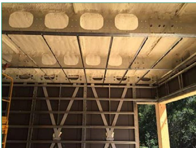
**Figure 2.** The home’s frame was designed by BONE Structure, a Canadian prefabricated home company. Photo courtesy SDI Insulation.
