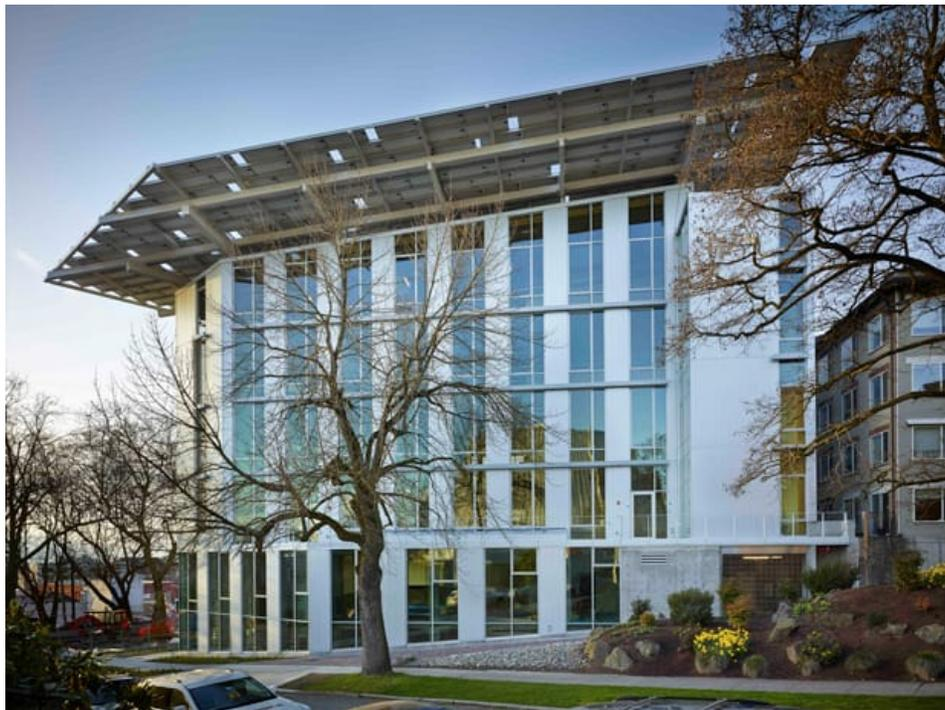
The wide roof overhang allowed the Bullitt Center in Seattle to capture enough solar energy to achieve net-positive energy. This six-story building uses 18 percent as much energy as a typical building this size. (Ben Benschneider)
